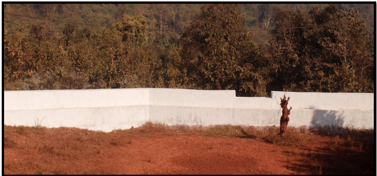
Photo showing check dams & Check weirs implementation within ML
