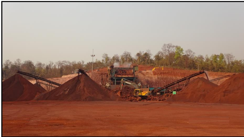
Photos showing dry fog implementations of various screens and crusher plant.
