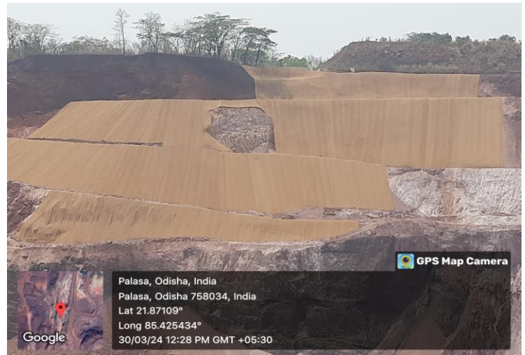
Photos showing Dump area plantations and worked out bench coirmat work
