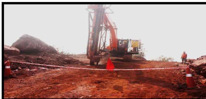
Photo Showing Excavate mounted Drilling Machine equipped with dust extractor & wet drilling mechanism
