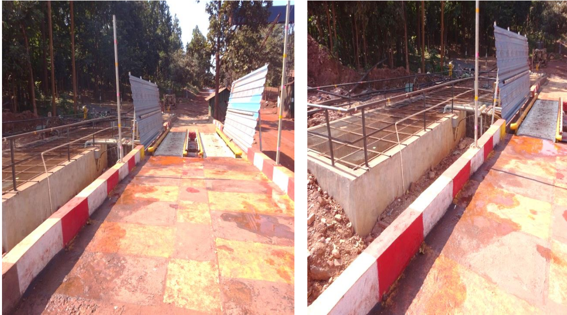
Photo showing the Mechanical wheel washing system at mines exit gate
